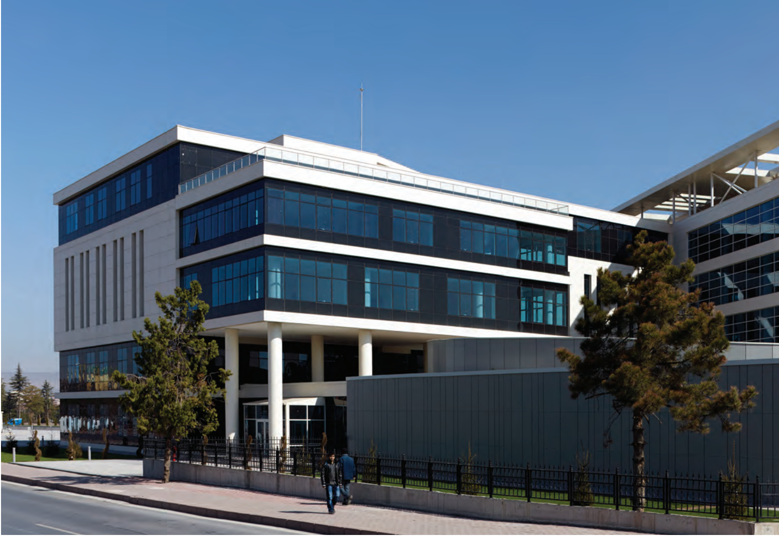
Kayseri Adliye Sarayı / Kayseri — Kalesinterflex 3mm Fit Mat Beyaz, 3mm Fit Mat Çimento Gri, 3mm Fit Mat Fildişi / Gizli Klipsli Sistem Kayseri Courthouse / Kayseri — Kalesinterflex 3mm Fit Matte White, 3mm Fit Matte Cement Grey, 3mm Fit Matte Ivory / Hidden Clips Fitted Facade System Mimar: Ven Mimarlık — Architect: Ven Architects
